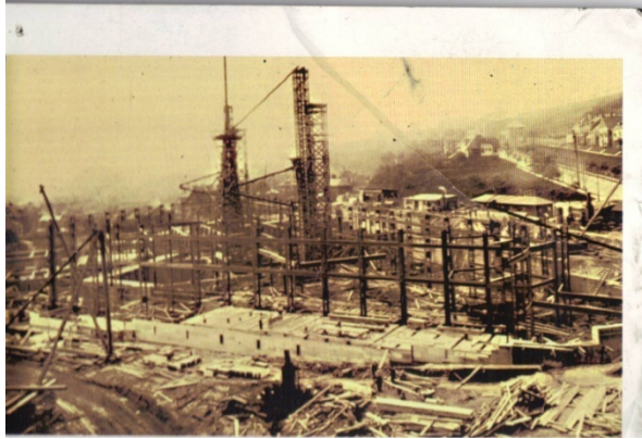
Construction of Schenley. Photo provided courtesy of James Hill
